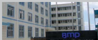
BMP ASIA INDUSTRIES (SHENZHEN) COMPANY LTD
